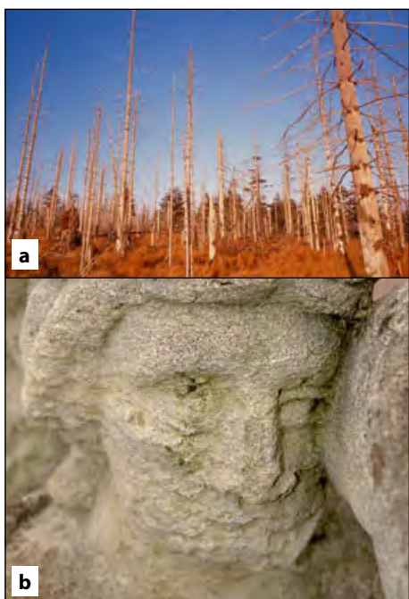
Figure 8.13 Acid deposition can a kill trees and fish in lakes and b react with limestone buildings to cause erosion.
