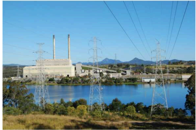
Figure 7.45 (a) Schematic of an electrostatic precipitator. Air is passed through grids of opposite charge. The first grid charges airborne particles, while the second attracts and collects them. (b) The dramatic effect of electrostatic precipitators is seen by the absence of smoke from this power plant. (credit b: modification of work by “Cmdalgleish”/Wikimedia Commons)
