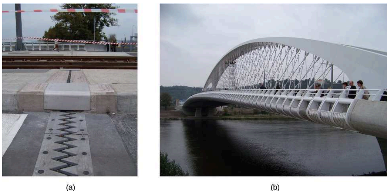
Figure 1.5 (a) Thermal expansion joints like these in the (b) Auckland Harbour Bridge in New Zealand allow bridges to change length without buckling. (credit: modification of works by “ŠJû”/Wikimedia Commons)
