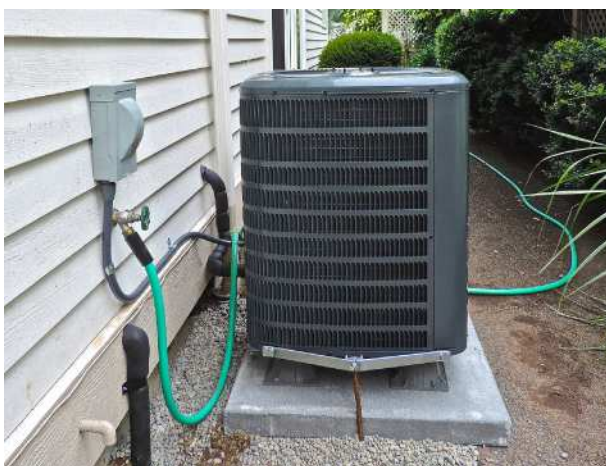
Figure 4.14 A photograph of a heat pump (large box) located outside a house. This heat pump is located in a warm climate area, like the southern United States, since it would be far too inefficient located in the northern half of the United States. (credit: modification of work by Peter Stevens)
