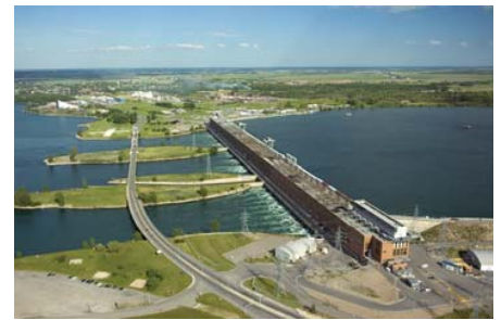
▲ Figure 9 Water as a primary energy resource. (a) A hydroelectric plant in Thailand. (b) A run-of-the-river plant in Canada.
