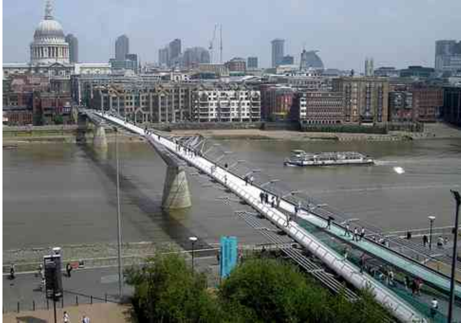
Figure 15.33 Initially when people crossed the London Millennium Footbridge, they experienced a swaying motion. People continuing to cross reinforced the oscillation's amplitude, thereby increasing the problematic swaying. (credit: Adrian Pingstone/Wikimedia Commons)
